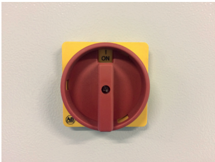
MAIN SWITCH – FIG. 10.26
