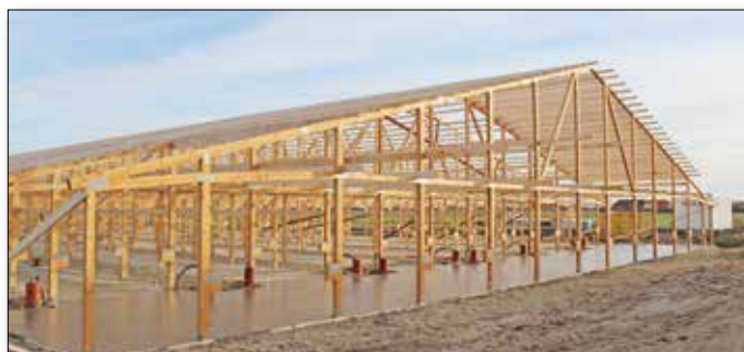
Ready for roof installation
