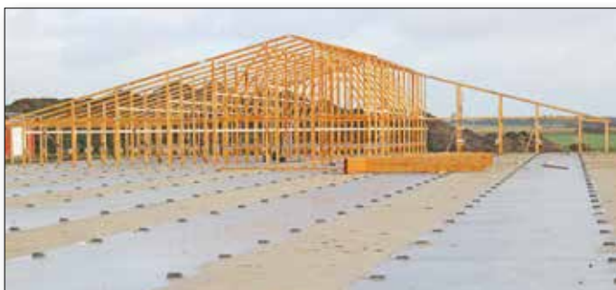
Installation of rafters
