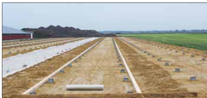
Casting the foundation
