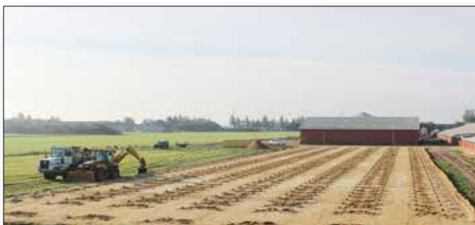
Base stones on sand ground
