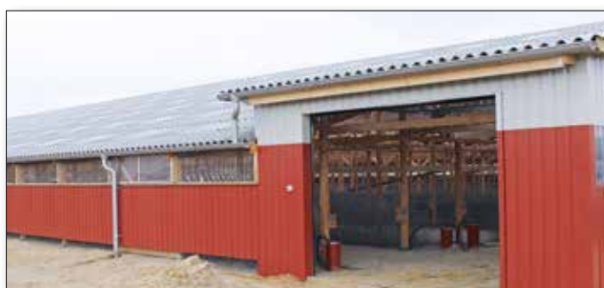
Ready for installation of manure gutters and water systems
