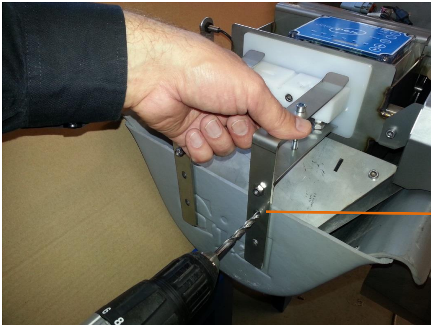
Fig. 4. Attachment of charging rails.
